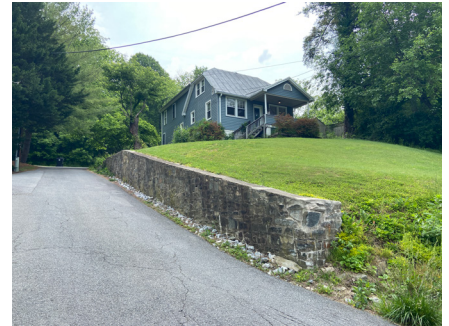
99. Maintain and repair existing site walls.
