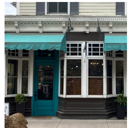
40 & 41. Commercial storefronts were constructed of wood and glass with the entrances recessed to protect patrons from the weather.
