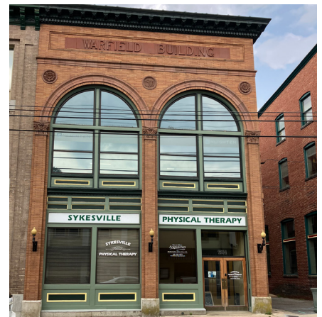
25. Masonry brick wall detail.
