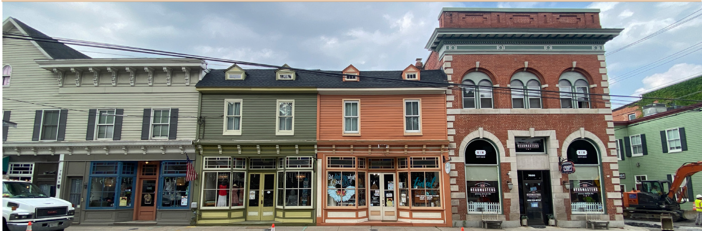
23. Masonry and wood exterior walls along Main Street.
