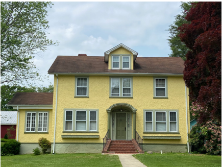
22. Front facade elements include foundation base and main walls with prominent front entry and steps.
