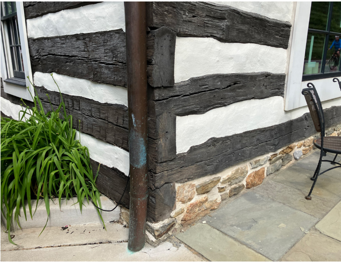
31. Recommended: Direct rainwater to underground piping.
