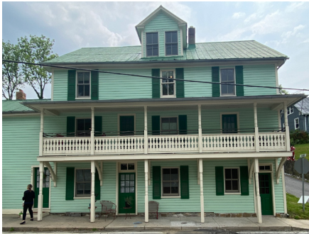
62. A two-story porch comprised of turned wood posts and balusters.
