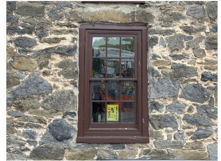
24. Masonry stone wall detail.
