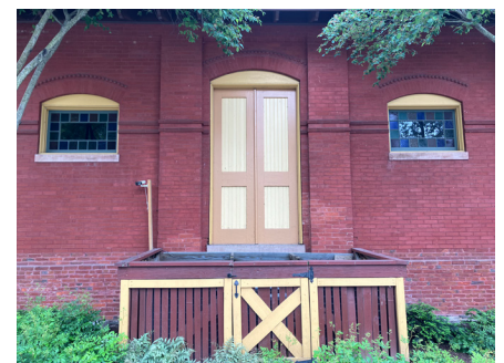
101. Screen trash enclosure.
