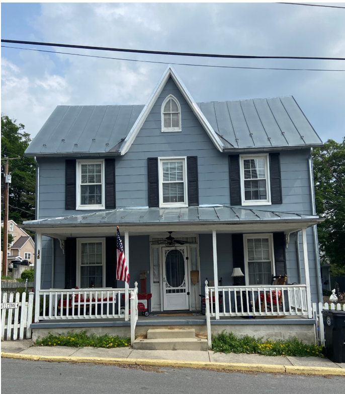
6. A Contributing building retains the historical significance of the district by maintaining its character defining features such as windows, roofing, and porch details.
