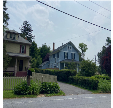
98. Driveways visually and physically connect many of the residential buildings in the historic district to the street.
