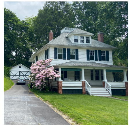
72. Accessory building (garage) on a residential property.
