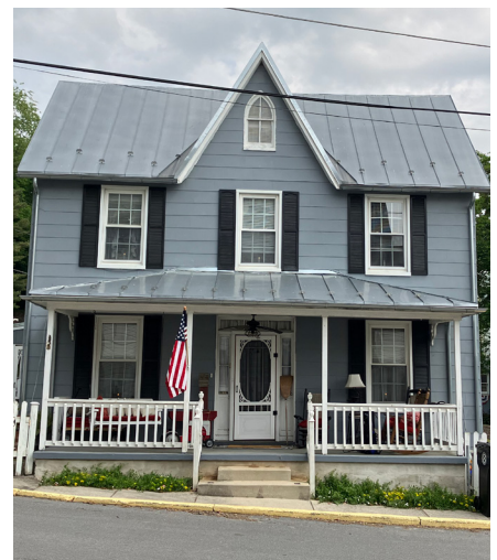
15. This historic metal roof is made up of hand-crimped metal pans.
