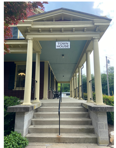
65. Porch with wood columns and iron railing.
