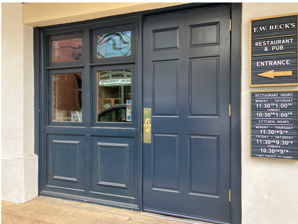
42. Main entry of a commercial storefront.
